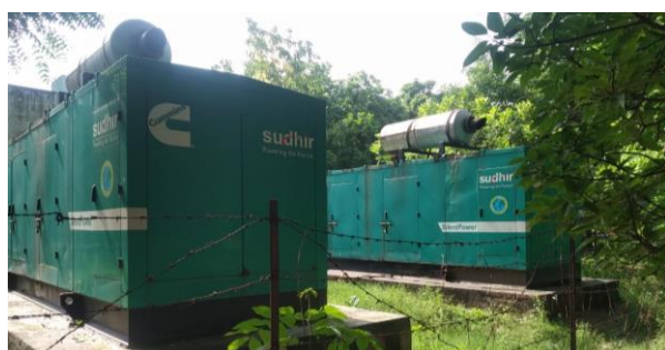
Figure 12: Diesel Generator Sets
