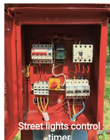
Figure 9: Timer Switches for controlling the 'On' duration of Street Lights
