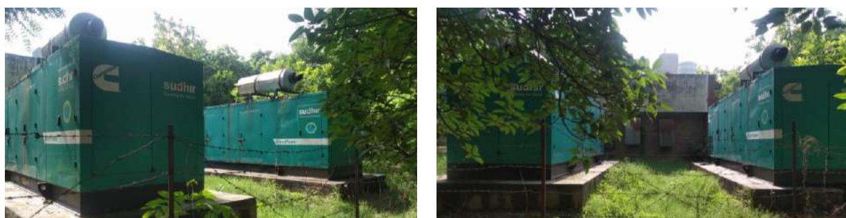
Figure 12: Diesel Generator Sets
