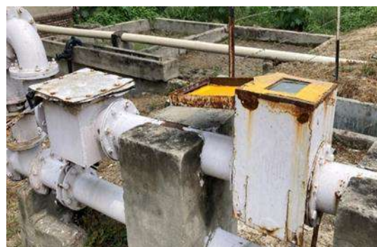
Figure 11: Ultrasonic Flow Meter at STP
