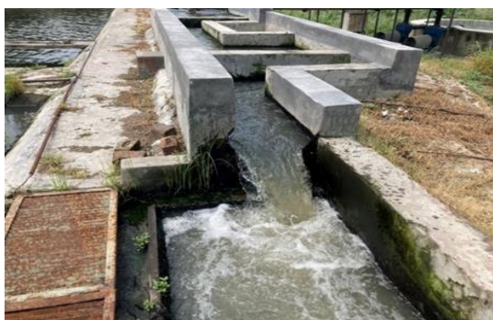
Figure 10: V-notch for Flow Measurement
