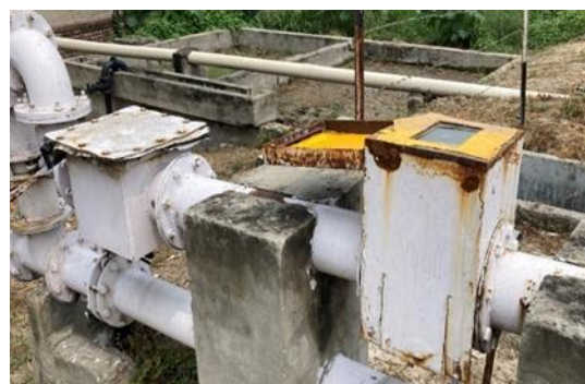
Figure 11: Ultrasonic Flow Meter at STP
